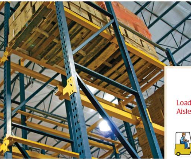
Pallets rest on rails within the bay.
